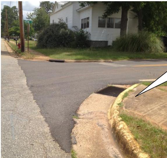
This photo demonstrates another section of the sidewalk which does not meet ADA and NACTO requirements located on the corner of Highland Avenue and Keene Street.
