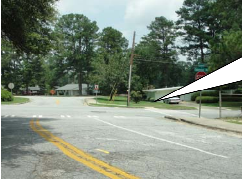
Intersection of Edgewood Rd and East Lindsey Dr. Sidewalk is abruptly cut of and provides no handicap access.
