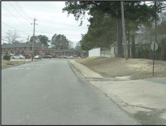
These photos demonstrate the current conditions of the sidewalks surrounding the school campus. Although some sidewalks are present, the conditions are inadequate in some sections; some have cracks and overgrown vegetation and almost all of them do not provide proper handicap access. As the pictures demonstrate, sidewalks do not have handicap accessible ramps, signs and proper pedestrian crossing signs.
